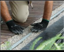
For outdoor applications, provide the appliance with drainage gravel for at least an additional 300 mm or an adequate drainage system.
