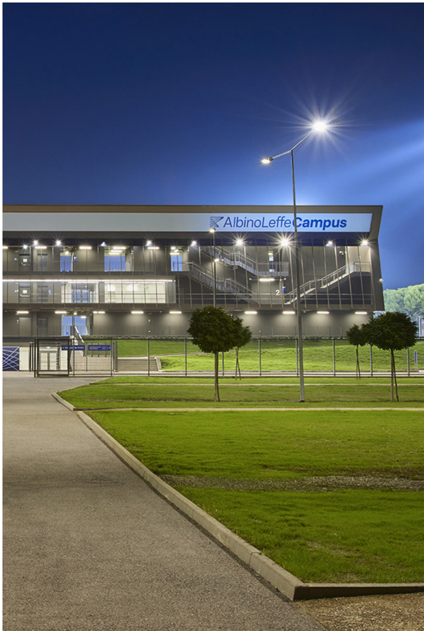
Albinoleffe stadium - Zanica - Italy
