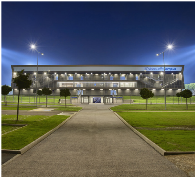
Albinoleffe stadium - Zanica - Italy
