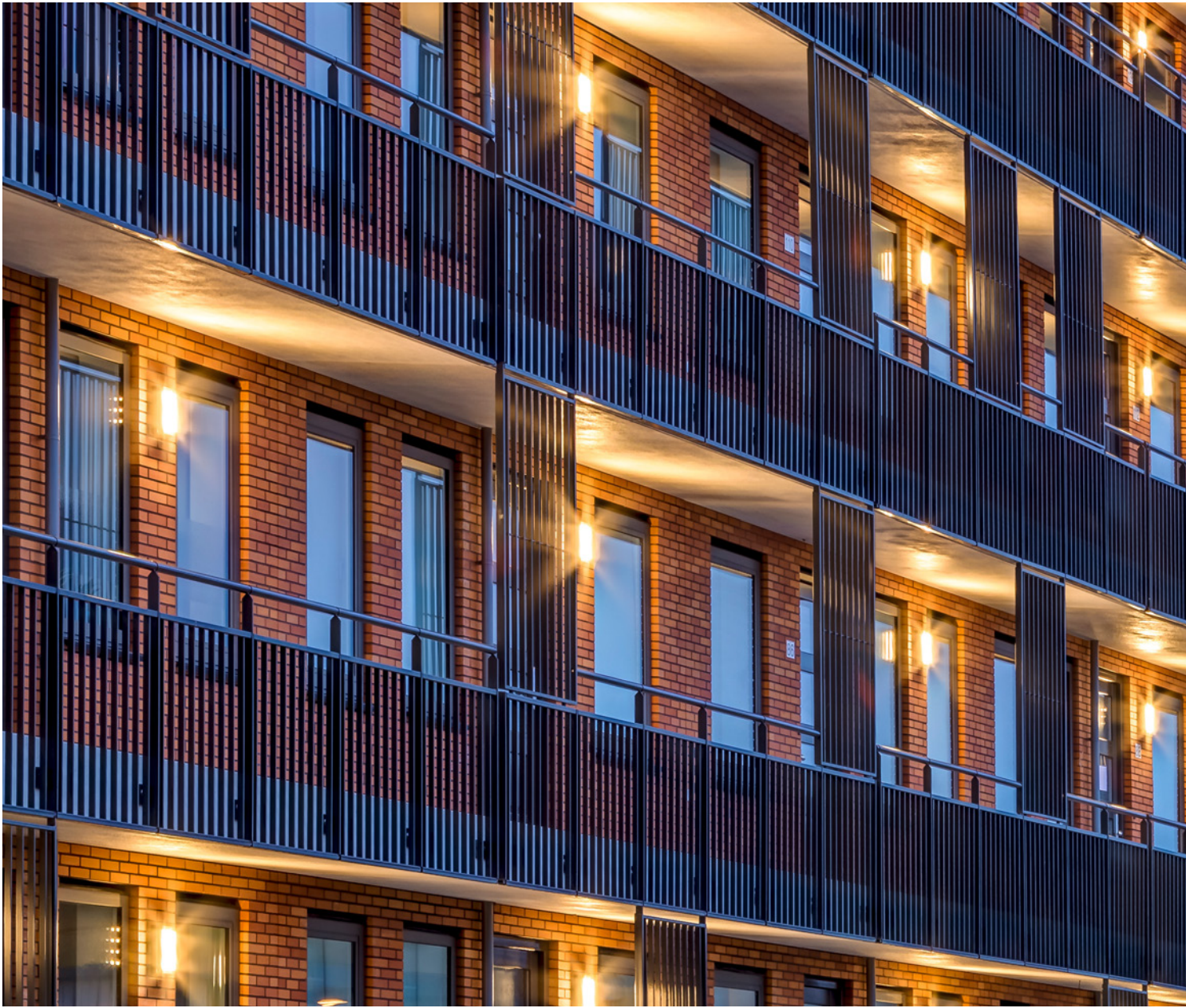
Residential Building De Bever - Heerhugowaard - Netherlands
