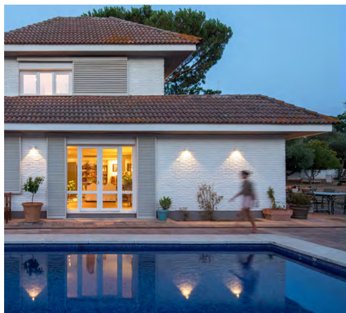
Private house - Andalusia - Spain
