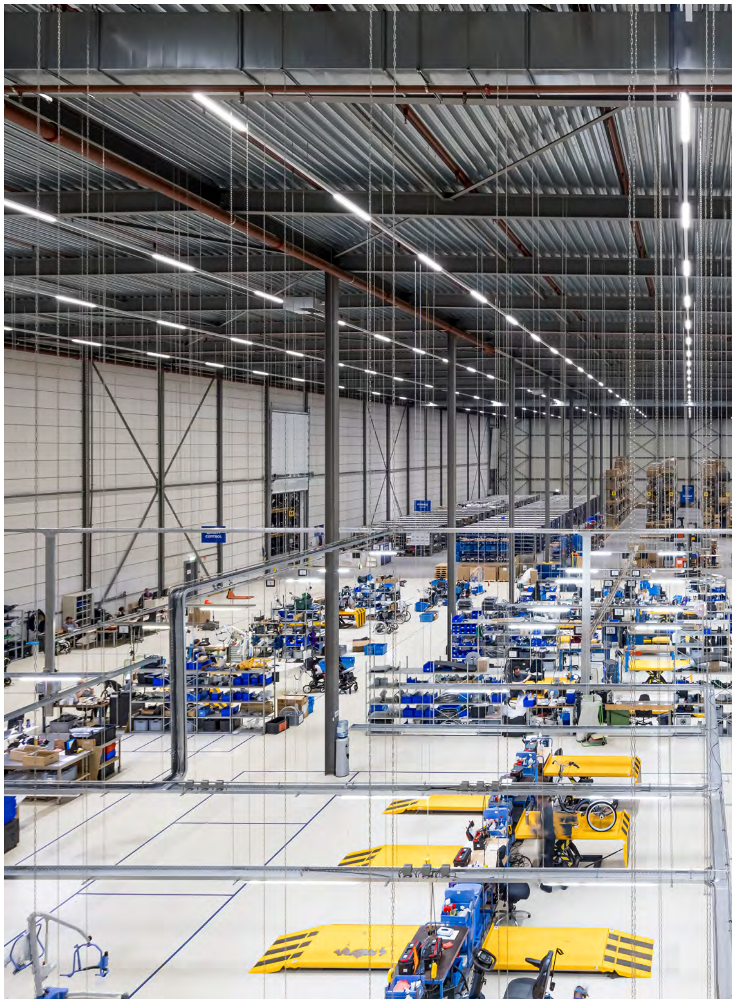
Welzorg distribution center - Raamsdonksveer - Netherlands
