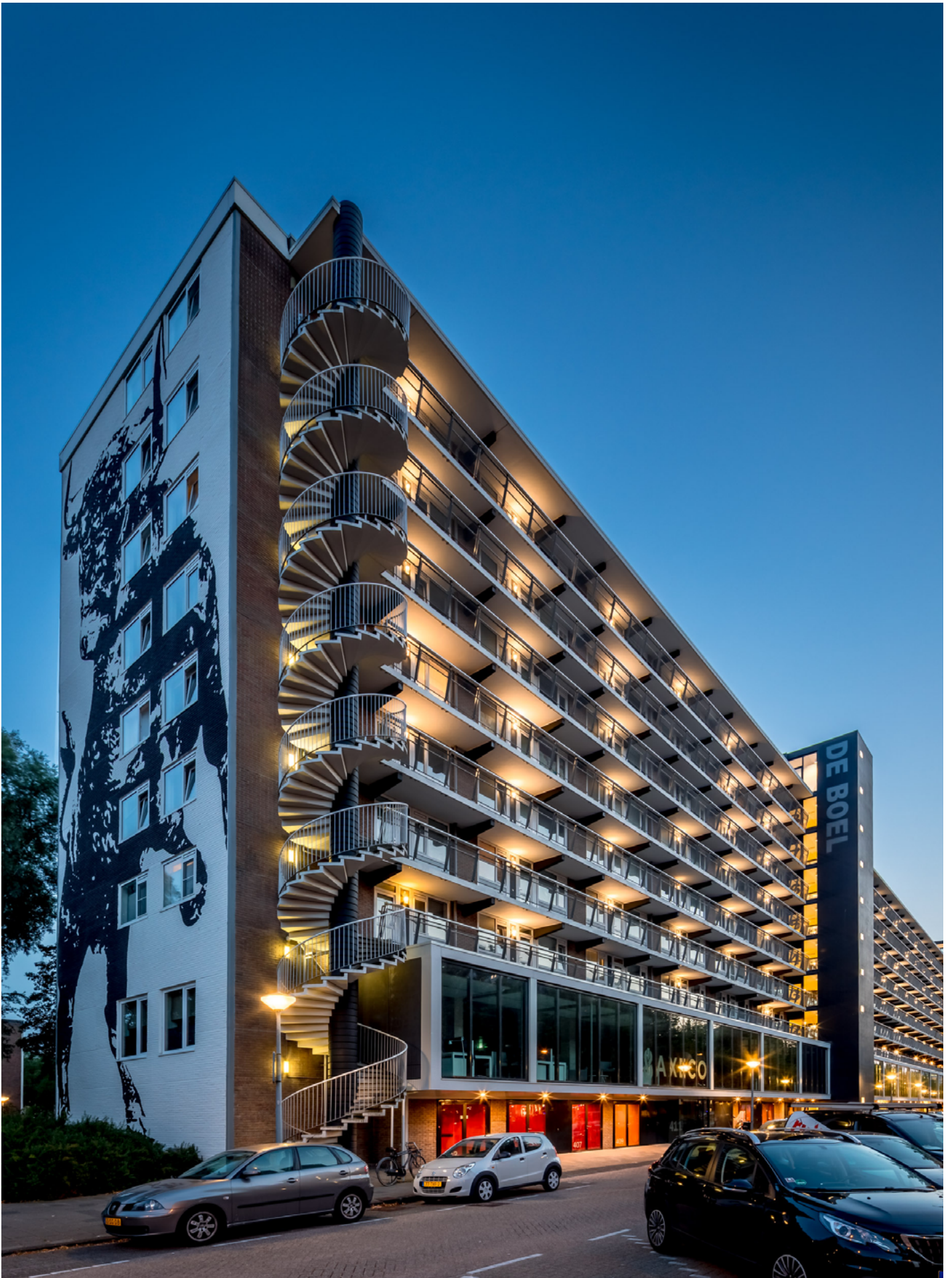
Apartment building De Boel | Amsterdam | Netherlands
