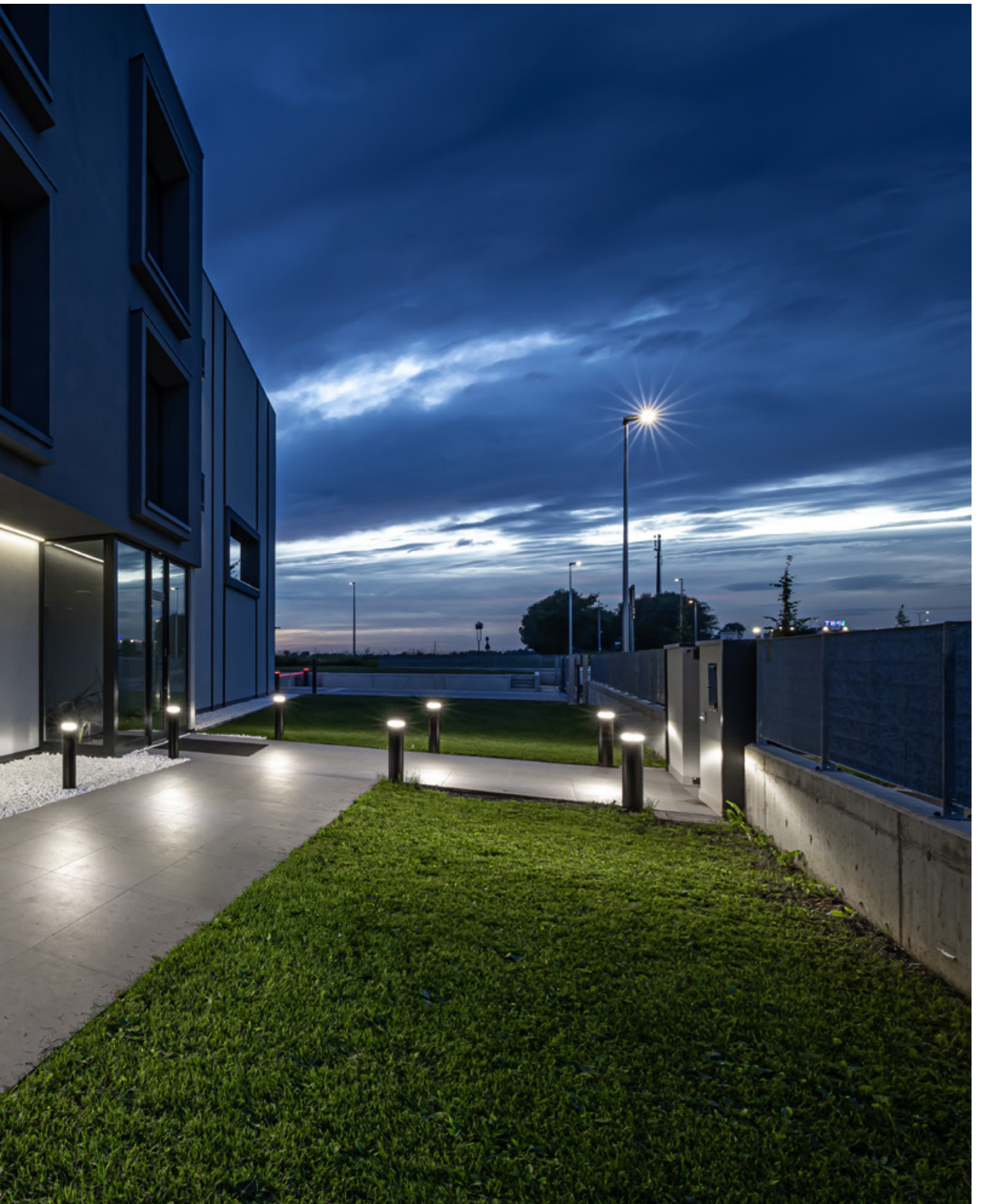
Marlegno headquarters | Bergamo | Italy
