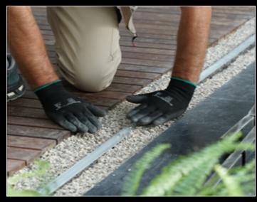
For outdoor applications, provide the appliance with drainage gravel for at least an additional 11.8 Inches or an adequate drainage system.
