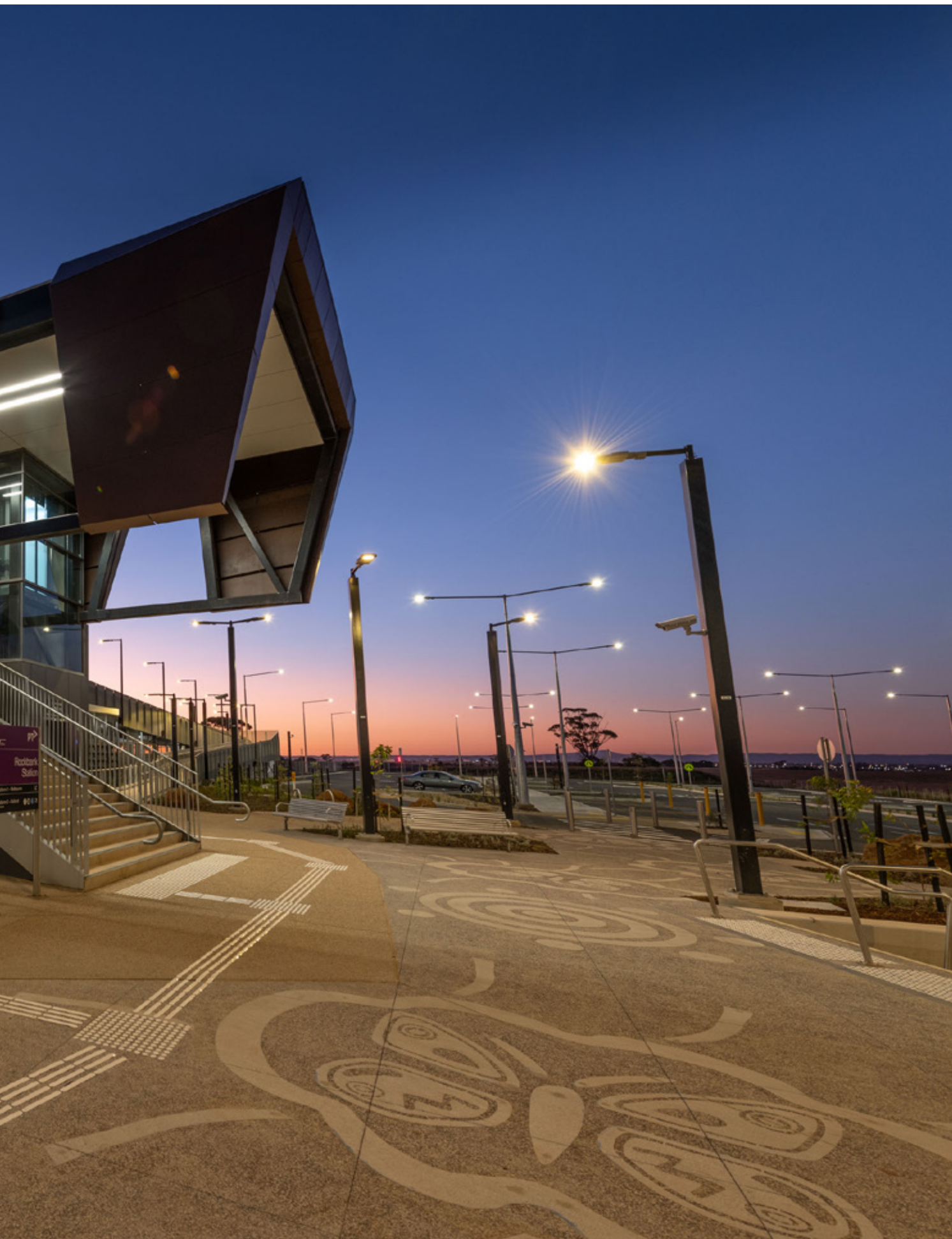
Train station Rockbank | Melbourne | Australia
