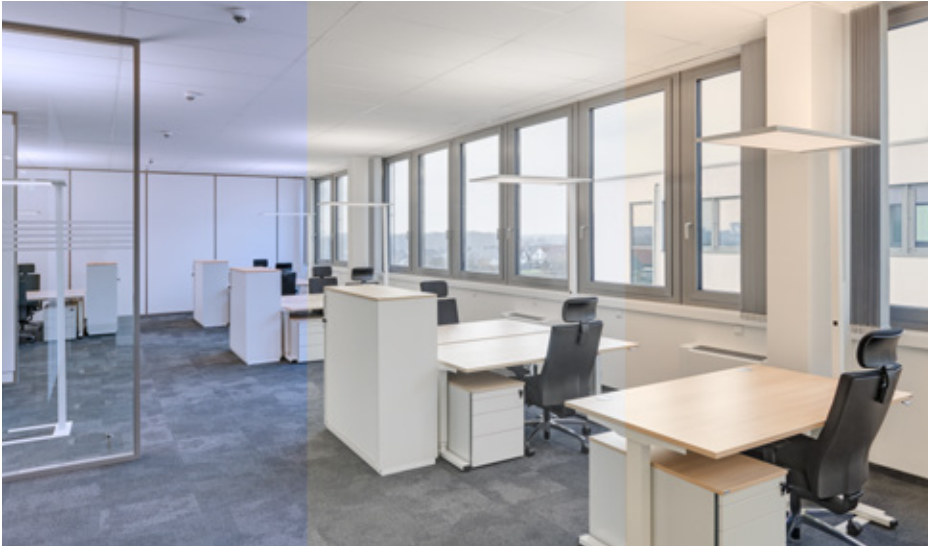
The HCL version reproduces the dynamic cycle of daylight in the indirect component, and varies the illuminance level and light colour between 2,700 K and 6,200 K depending on the time of day
