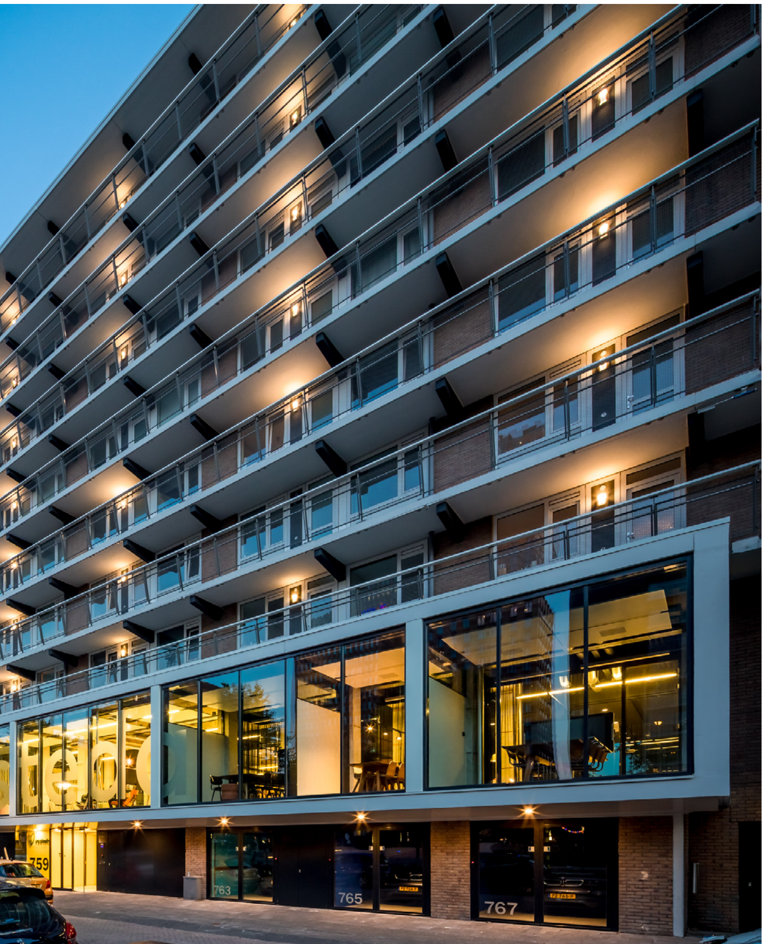
Apartment building De Boel | Amsterdam | Netherlands
