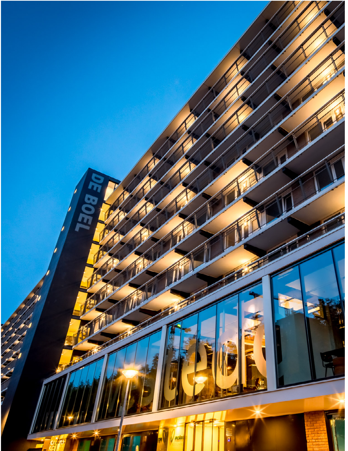
Apartment building De Boel | Amsterdam | Netherlands
